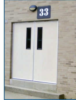
Exterior door with number on building
